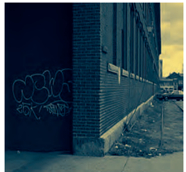
Signs of urban decay
